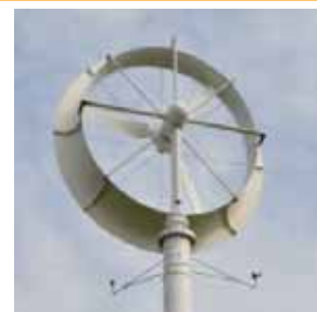
3 kW lens windmill (single machine), Kyushu University Ito Campus installed, and about 10 other turbines (independent system)
