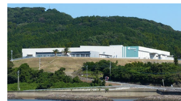
FI plant in Matsuura, Nagasaki, where the company was founded. Manufacturing roofing materials with the latest equipment
